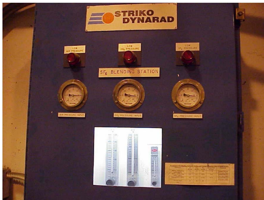
Figure 4 Cover gas blending station.
